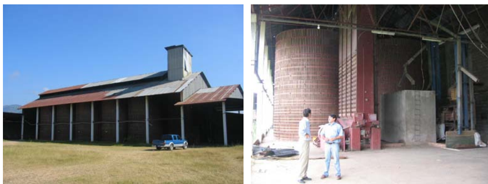
Images of the grain drying installations of COOPACYL in Yoro.
